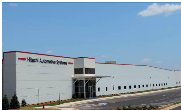
Hitachi Automotive Systems Americas, Inc. Georgia Plant Third Production Facility
